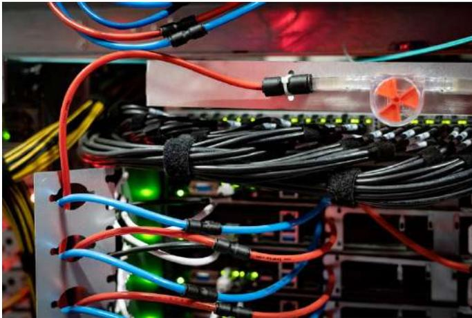
OVHcloud water cooling; blue pipes pump cooled liquid to the CPU and red pipes capture heat for transfer.
